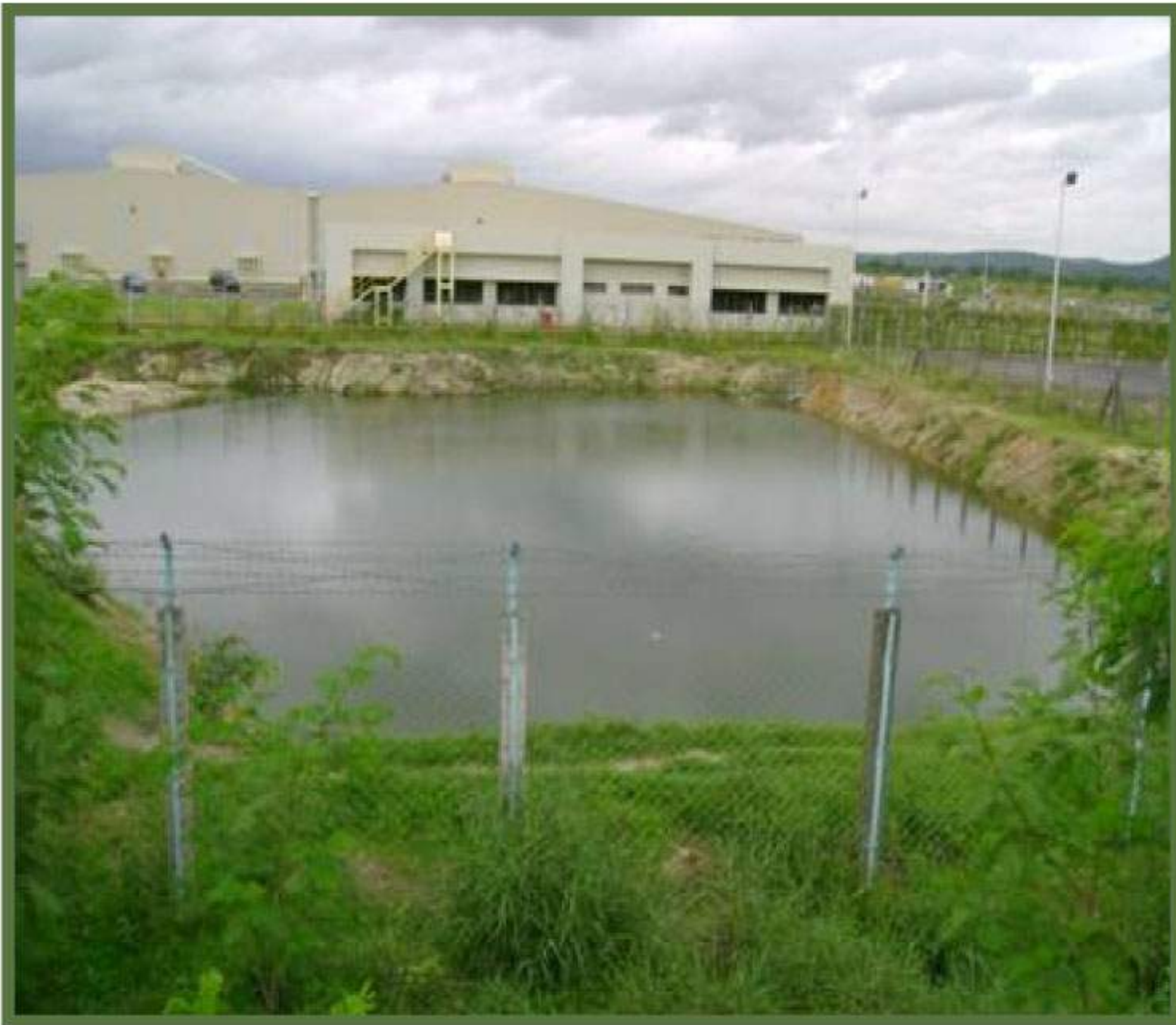
Fig 6.6: Rain Water Harvesting Pond
