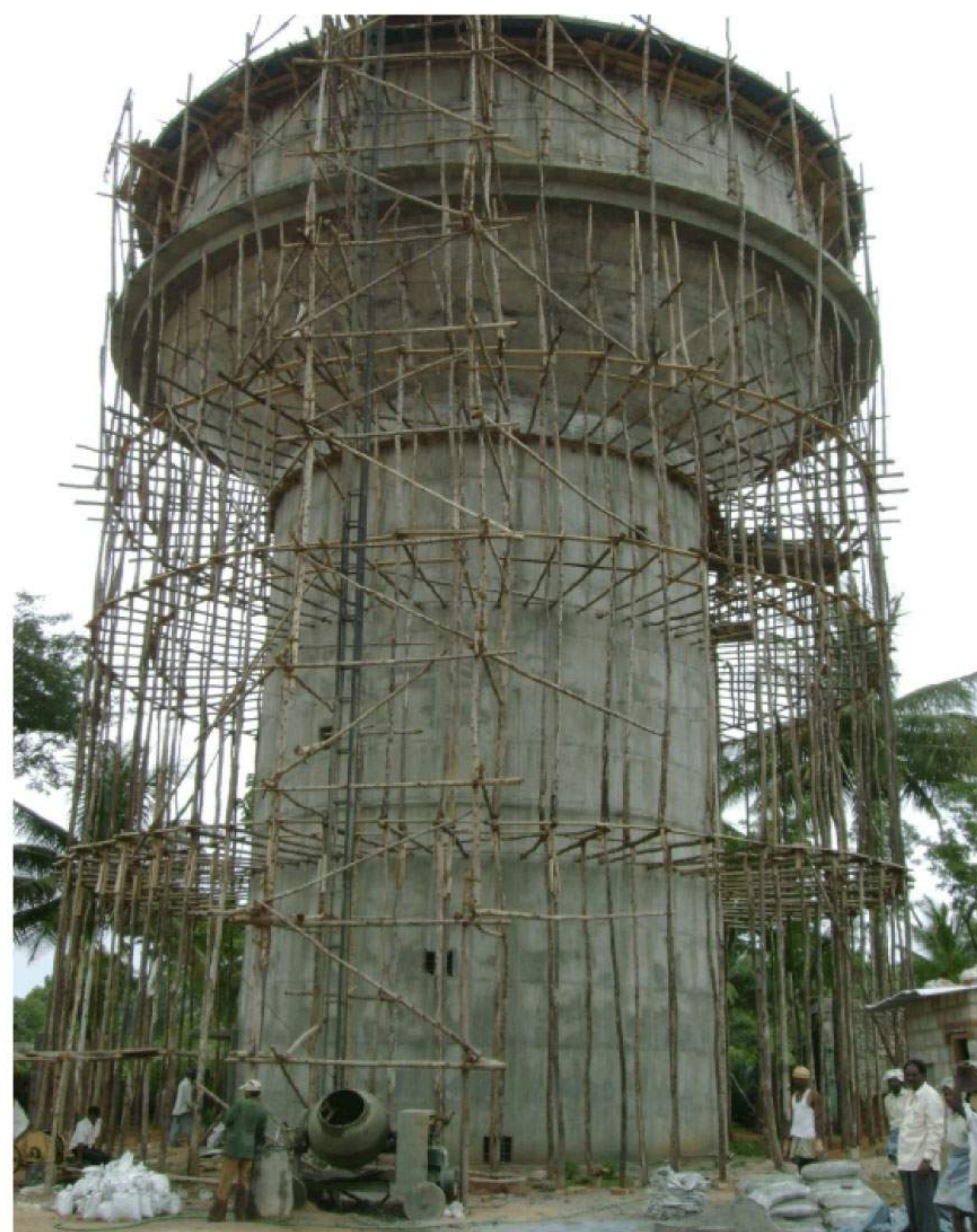
Fig 10.1: Construction of Water Tank
