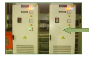
Fig 5.5: VFD installed at Paint Shop to optimize the electricity consumption ultimately yielding 12% reduction
