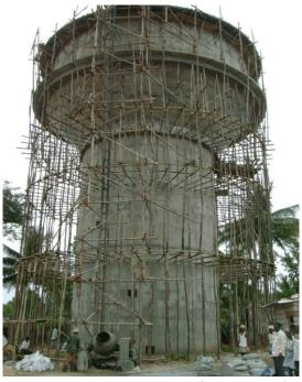
Fig 10.1: Construction of Water Tank
