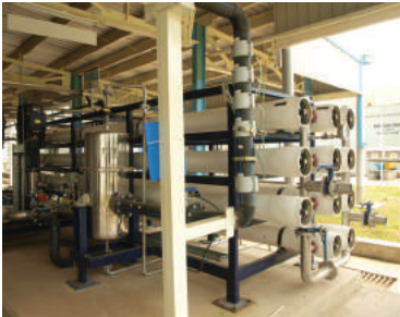
RO and MBR Installation at TKM premises
